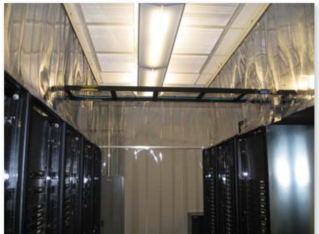
Aisle Containment Curtains easily conform to overhead obstacles
